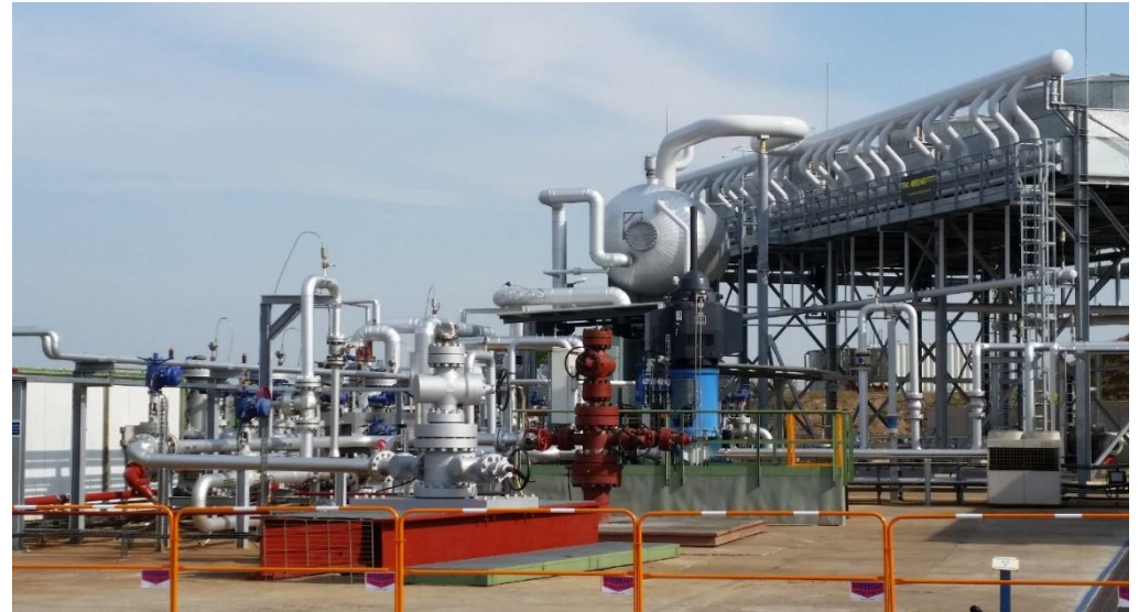
II. ORC unit : heat/power conversion
